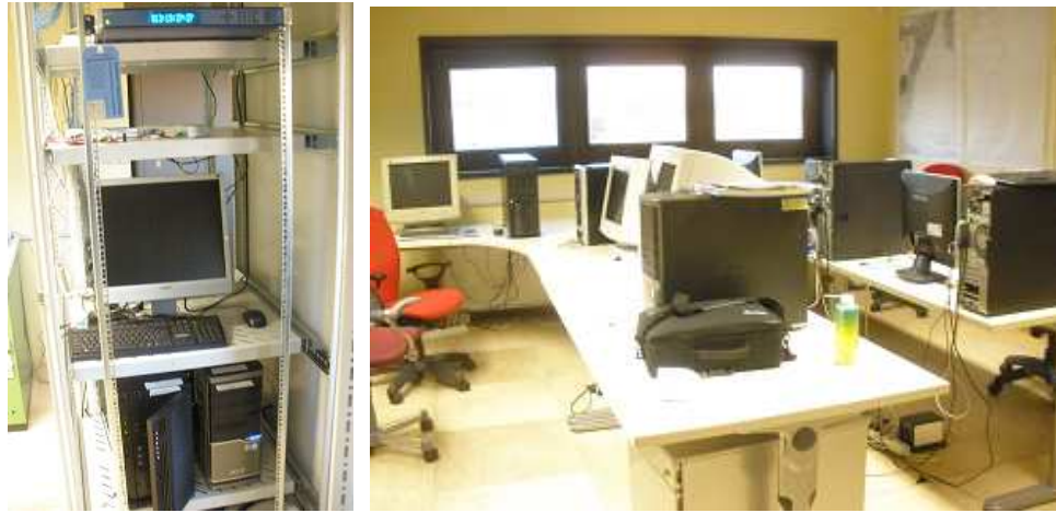
Figure 4.5. Telemetry rack for acoustic sensors (left), and data archiving and monitoring room at the INFN shore Laboratory.
