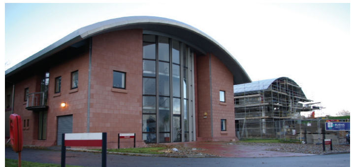
Oceanlab II is currently under construction and will be commissioned in May 2009.
