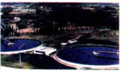
Station d'epuration - Sousse
