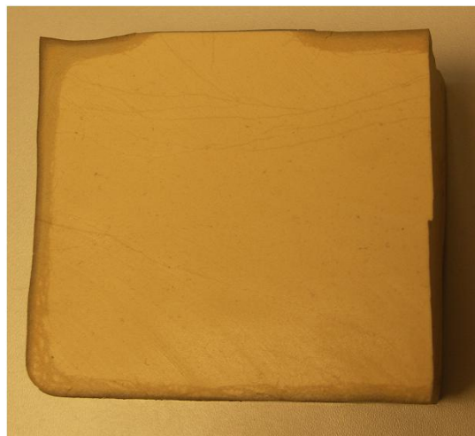
Figure 121: superficial degradation of 25 years exposed syntactic foam material (10cm*10cm block)
