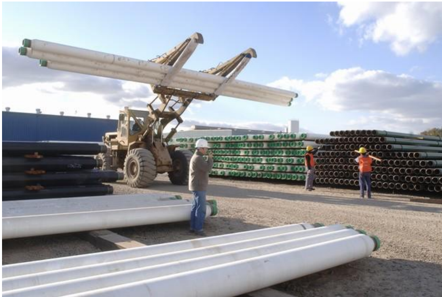
Figure 15 : GSPP insulated pipelines courtesy Socotherm
