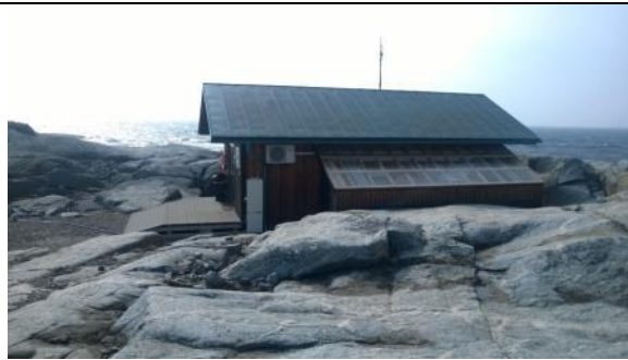
Utö measuring cabin outside
