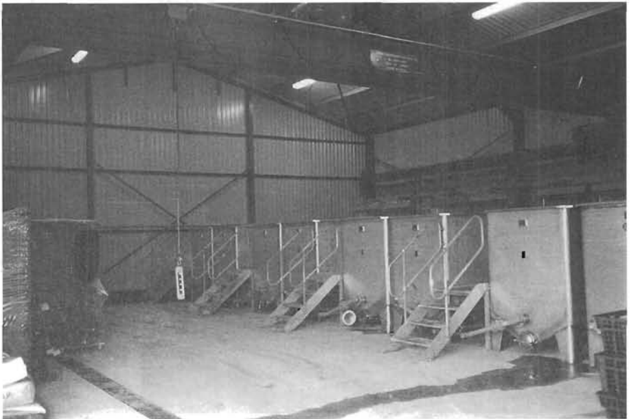
Figure 4: Purification plant at Kings Lynn
