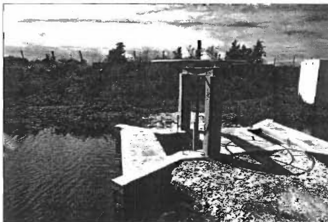
▼ Flood-gate regulating the water level of a rearing pond in the Gironde region, France (Photo Serge Lucas).
