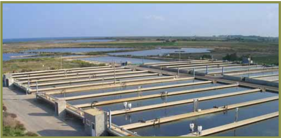
Figure 1: A general view of Maribrin's tanks and the filter that is used (Photo STM aquatrade)
