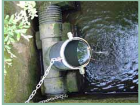
Figure 6: Simple water-level control mechanism.
