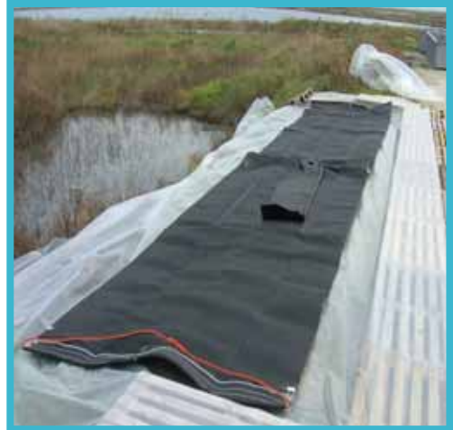
Figure 7: The geotube before filling
