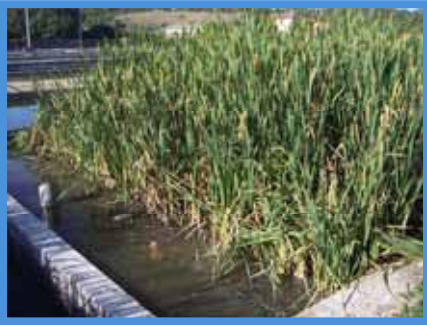
Figure 11 and 12: Horizontal wetland system and vertical wetland systems
