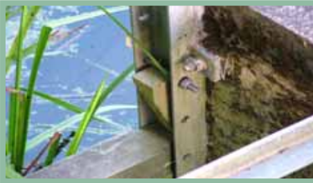
Figure 7: Sluice systems to maintain water levels. Simplest is best (photo G. Proffitt)
