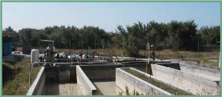
Figure 2: Settlement tank (photo STM aquatrade)
