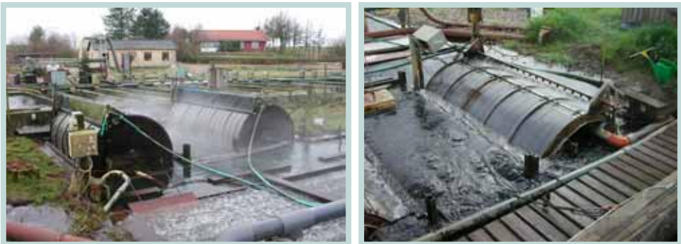
Figure 4: Microsieve drum filters. The photographs show the sieves operating under two conditions. (A) the sieves are set relatively high, with about 30% immersion. (B) the current position, with sieves 80% immersed. See Figure 1 for the sieve drum filter location.
