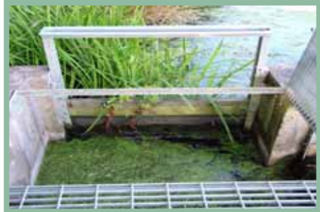
Figure 6: Simple water-level control mechanism.
