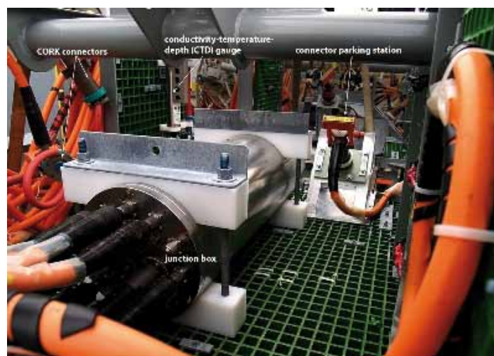
Fig.6 - Connection of the Neptune Canada junction box
