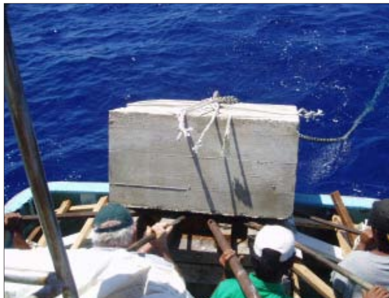
Mooring the deadweight (2 t concrete block)
