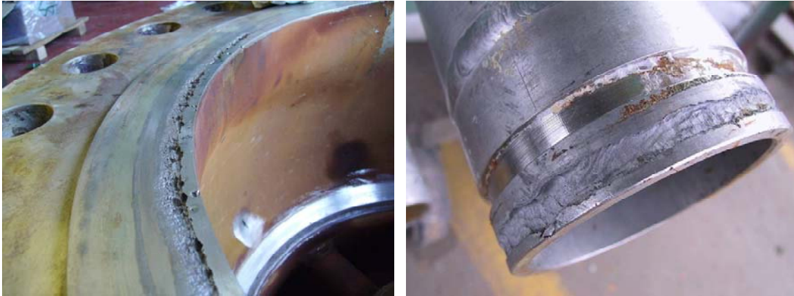
Figure 9 : (a) Crevice corrosion of a cast superduplex stainless steel at gasket location, (b) crevice corrosion of a wrought superduplex stainless steel at a “Victaulic-type” connection.
