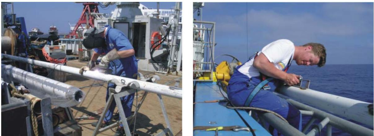
Figure 7.1 (a) Leon Wuis welds outrigger probe thermal holders on core tube. (b) Tomas Feseker attaches a thermal probe to one of the probe holders.
