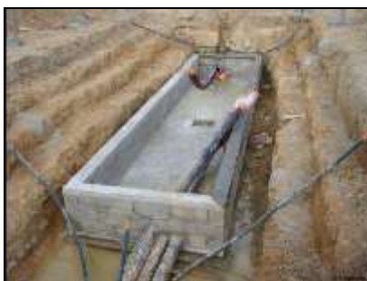
Figure 20 Junction box (source: RTE)
