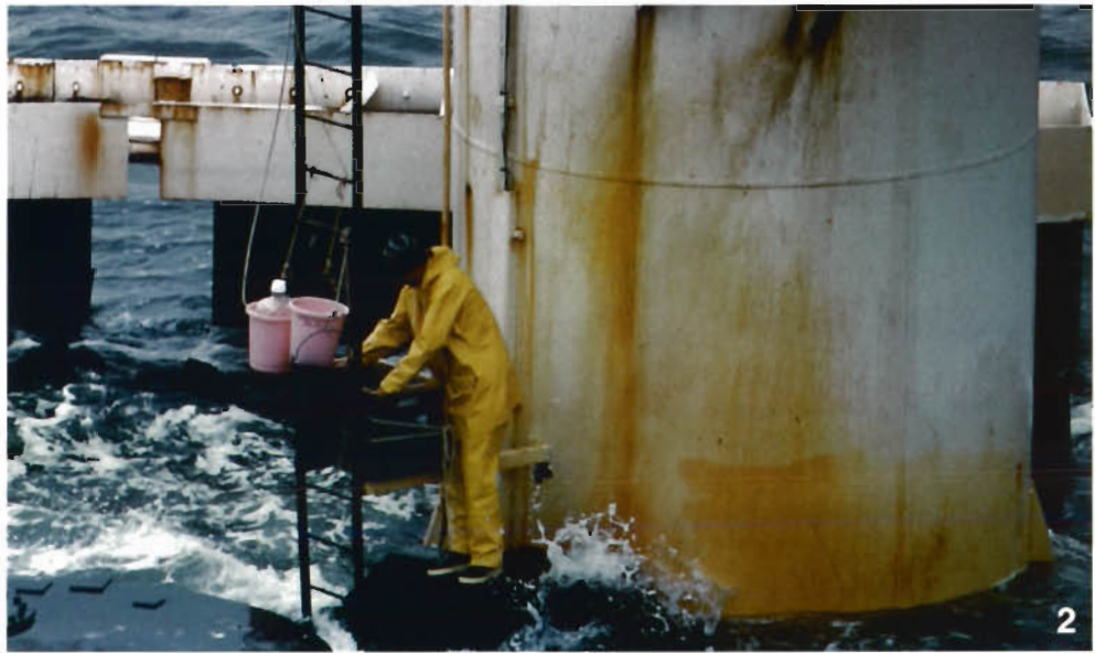
Fig. 2. Sampling of surface water from the pier of Antifer harbor
