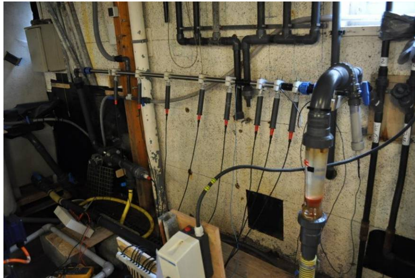
Figure 3: Schematic drawing and photograph of the 2 m-long monitored superduplex stainless steel pipe
