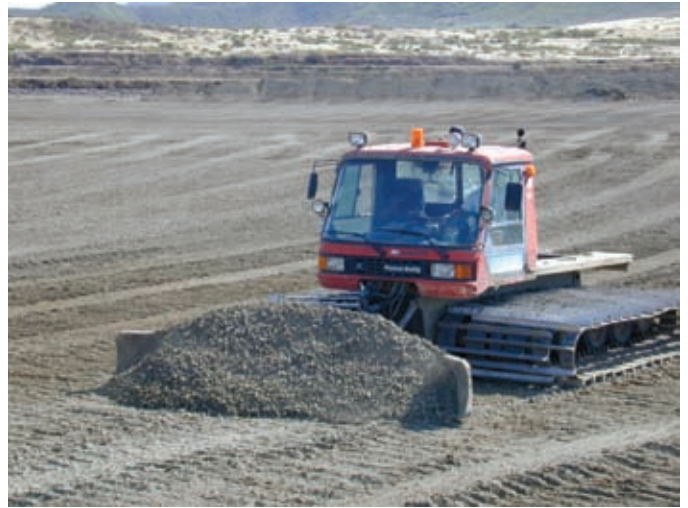
Fig. 6. Soil work with a snowplow.
