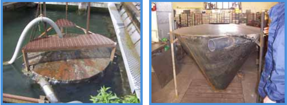
Figure 5 and 6: Thickening tanks
