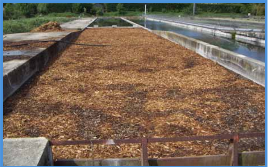
Figure 15: Current sludge storage system: settling tank with wood shavings
