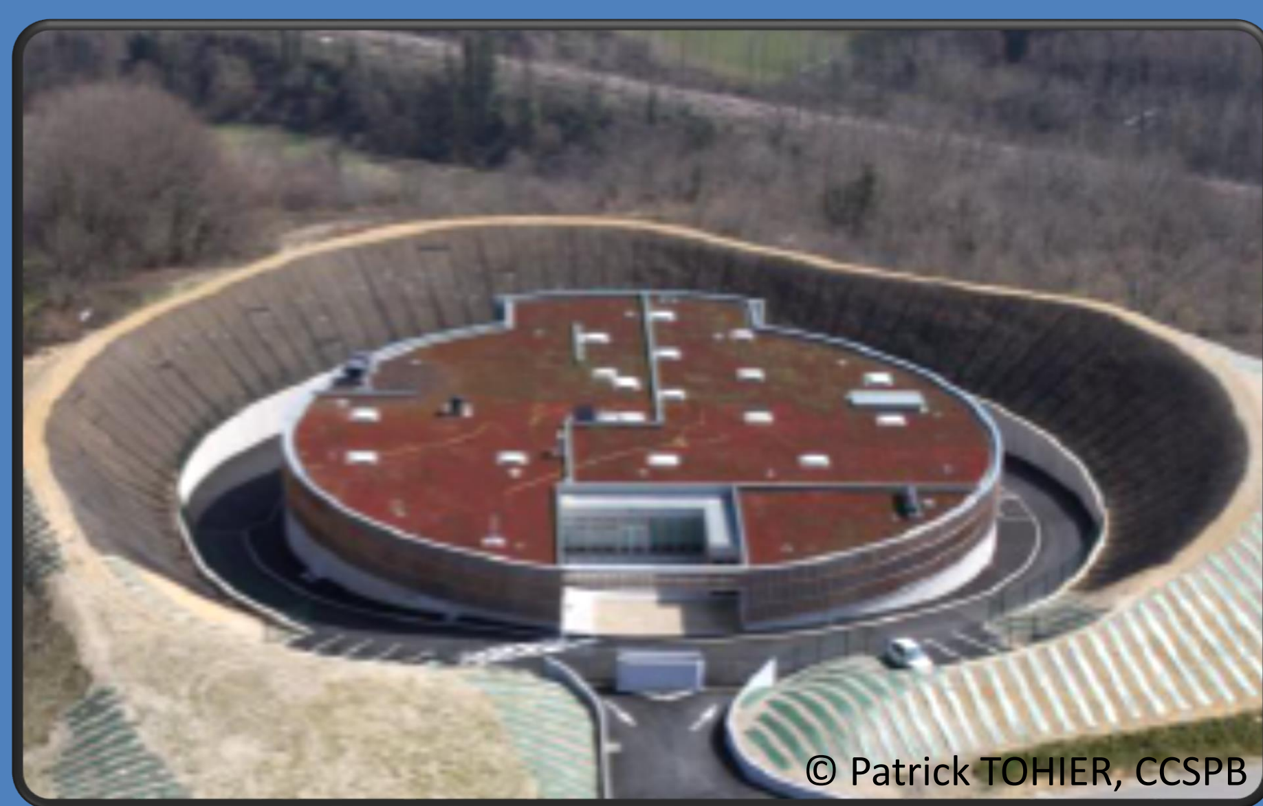
Fig.1: Water Treatment Plant (WTP)
