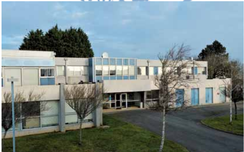
The Cersat building at the Ifremer Centre in Brittany
