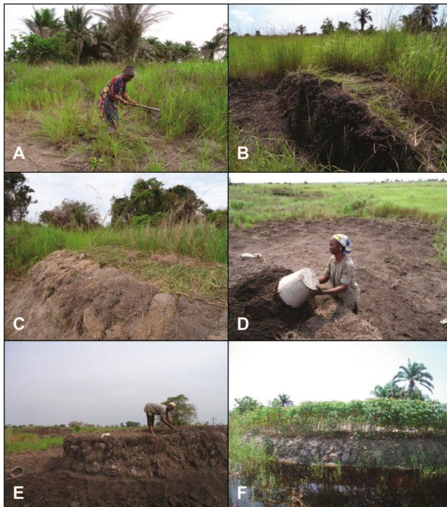
Figure 4. Construction of RF in the floodplain around Mossaka. (A) Grass and soil clumps are hoed from the area surrounding the new field; (B,C) Root-bound soil clumps are oriented outward, the grass tops are oriented inward; (D) Vegetation-free topsoil is added to cover the field; (E,F) The new field is soon planted with manioc, the major crop. All photos © M. Comptour.
