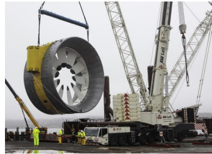
Figure 4 – Assembly of OpenHydro turbine ©OpenHydro
