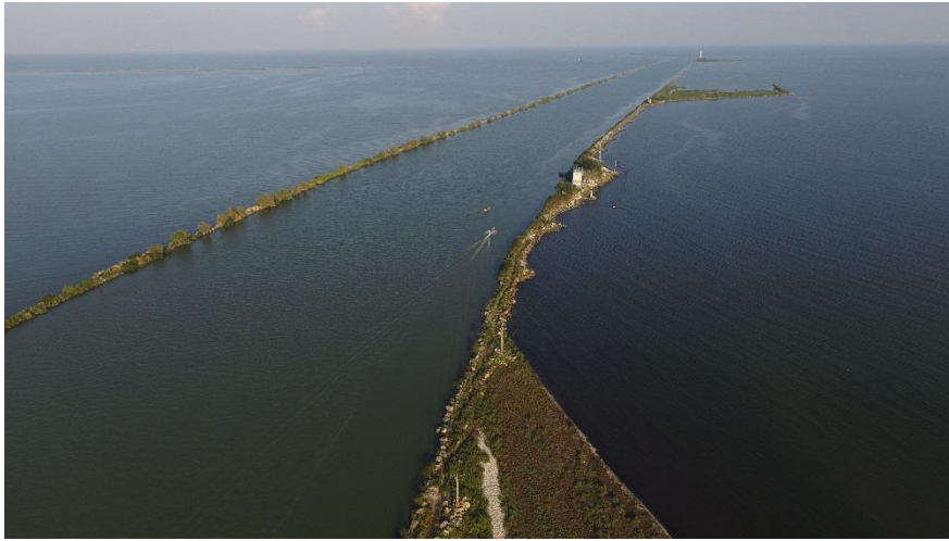
Figure. 8. Protection dikes of Sulina channel (Danube branch) (source: NIMRD database)
