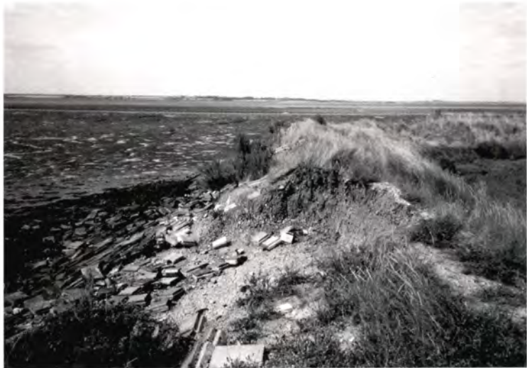
Plate 1 Erosion of fronting saltmarsh has exposed many seawalls to direct wave impact leading to structural damage and subsequent flooding and erosion.
