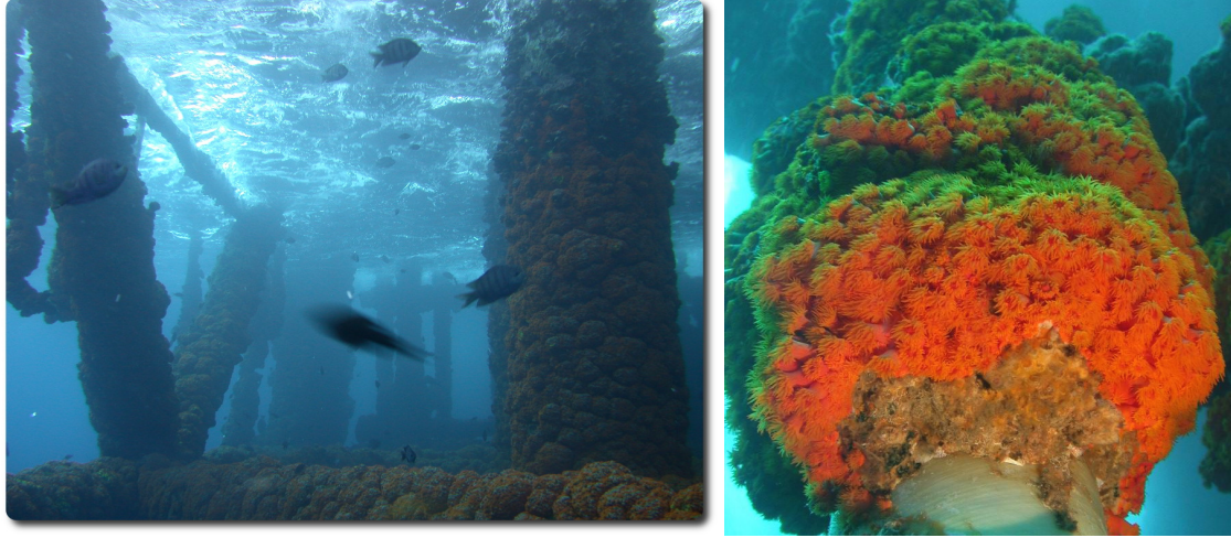
Figure 2: Illustration of corals colonisation on a jacket of marine platform in West Africa, with a tubular bracing structure of 0.2 to 2m diameter.
