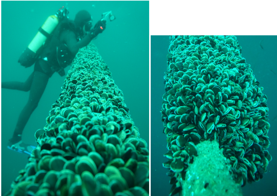
Figure 1: Illustration of mussel colonisation on a mooring line (West coast of France on a 0.1m diameter mooring line at 10m depth) [13].
