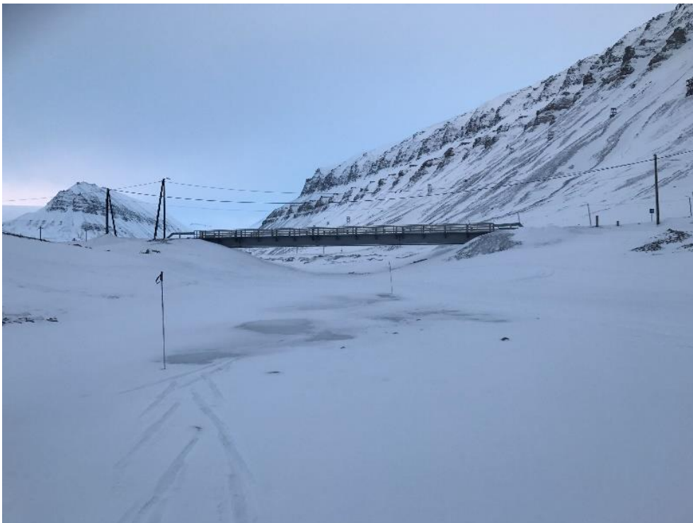
Figure S1.a7-1. Small and medium-size, not cracked icings at Longyearelva below the bridge over the Road 501 (03.05.2017, location a7 in Table S1). Photo: © Anatoly Sinitsyn.
