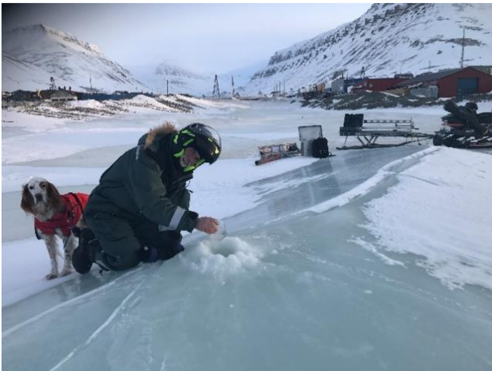
Figure S1.a1-4. Small, cracked "mound" icing at Longyearelva below the bridge across the Road 600 (18.04.2017, location a1 in Table S1), drilling revealed water at artesian pressure. The water had distinct taste and smell of diesel. Photo: © Anatoly Sinitsyn.
