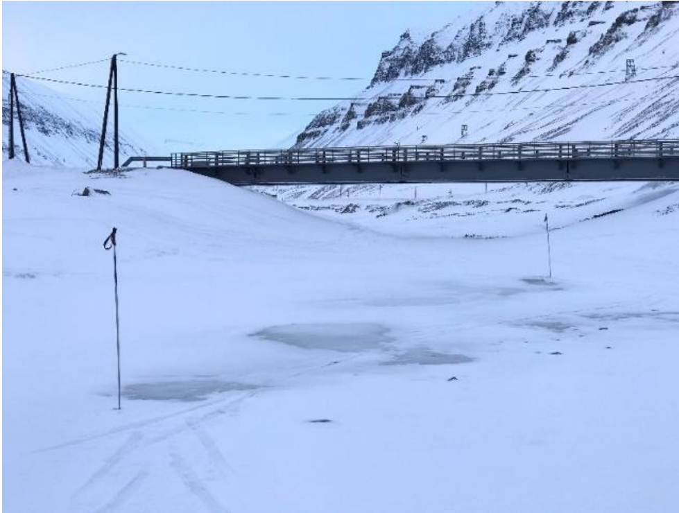
Figure S1.a7-2. Small and medium-size, not cracked icings at Longyearelva below the bridge over the Road 501 (03.05.2017, location a7 in Table S1). Photo: © Anatoly Sinitsyn.
