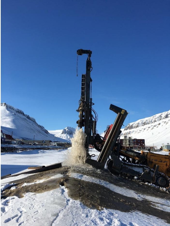
Figure S1.a11-3. Emergence of water at artesian pressure when drilling through an icing in Elvesletta (23.04.2018, location a11 in Table 1). Photo: © Marit Pedersen/Ramboll AS.
