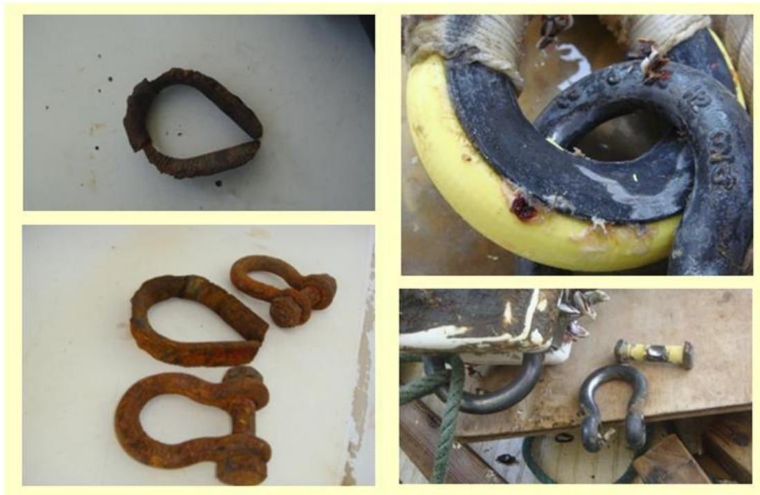
Photo 8: Comparison between metal pieces after 2 years in the sea protected and unprotected by anodes.
