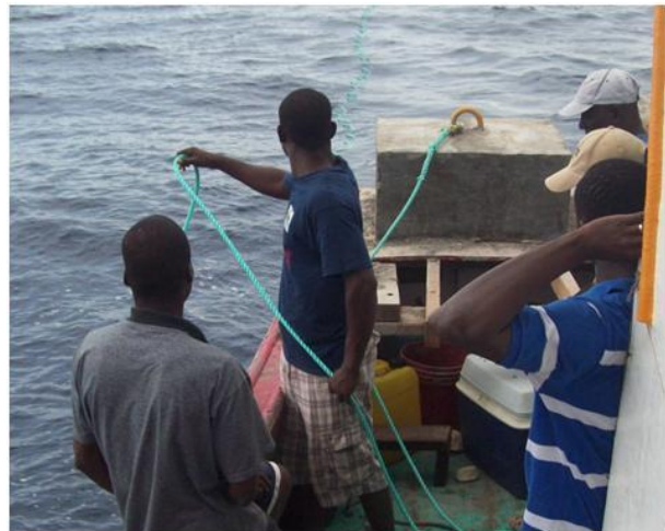
Photo 20: A makeshift table raises the block slightly above the transom.
