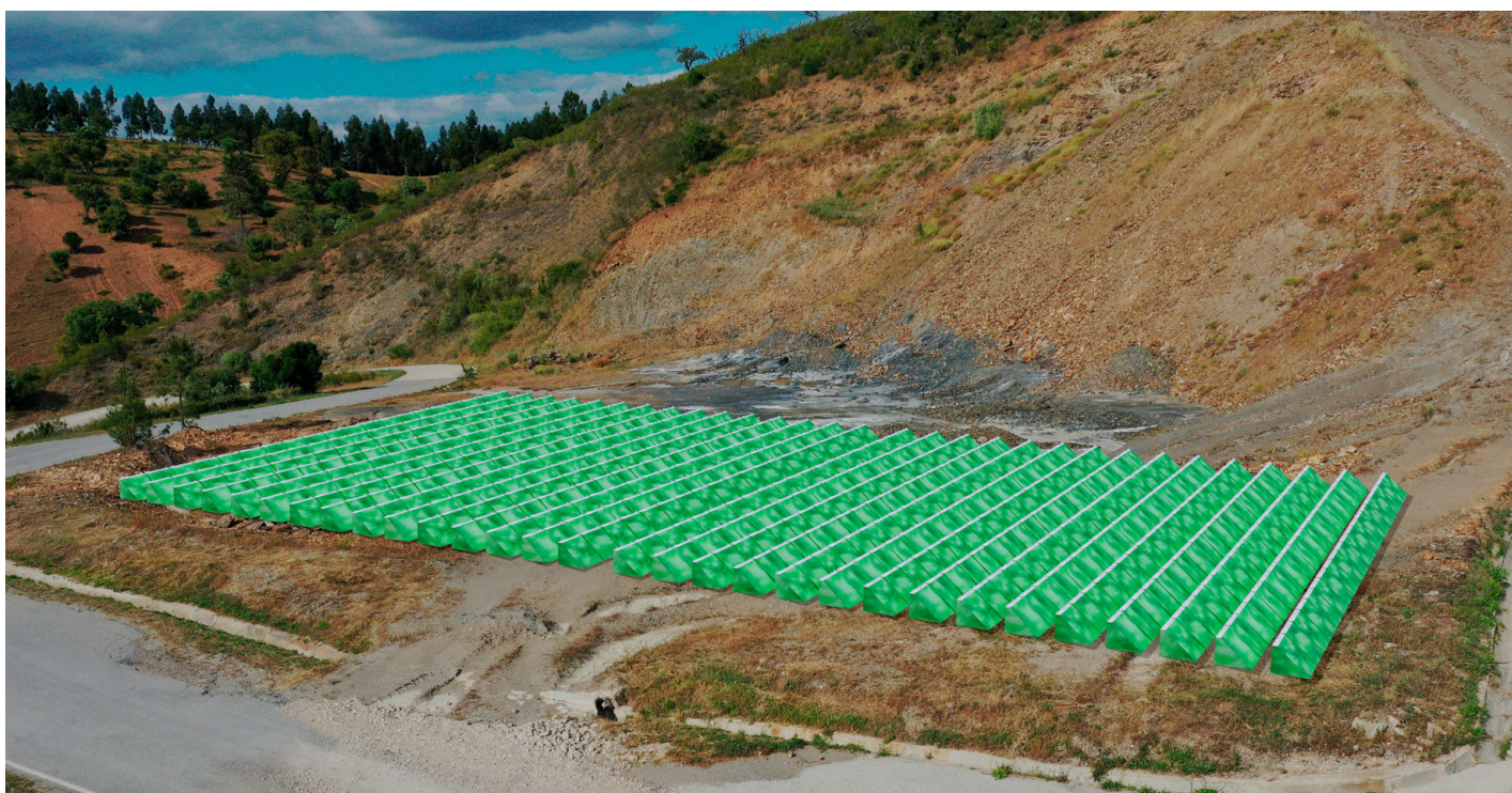
The ALGAMATER Project Green Dune photobioreactor installation in Algarve, Portugal. This technology is being further developed within the RHE-MEDIation Project
